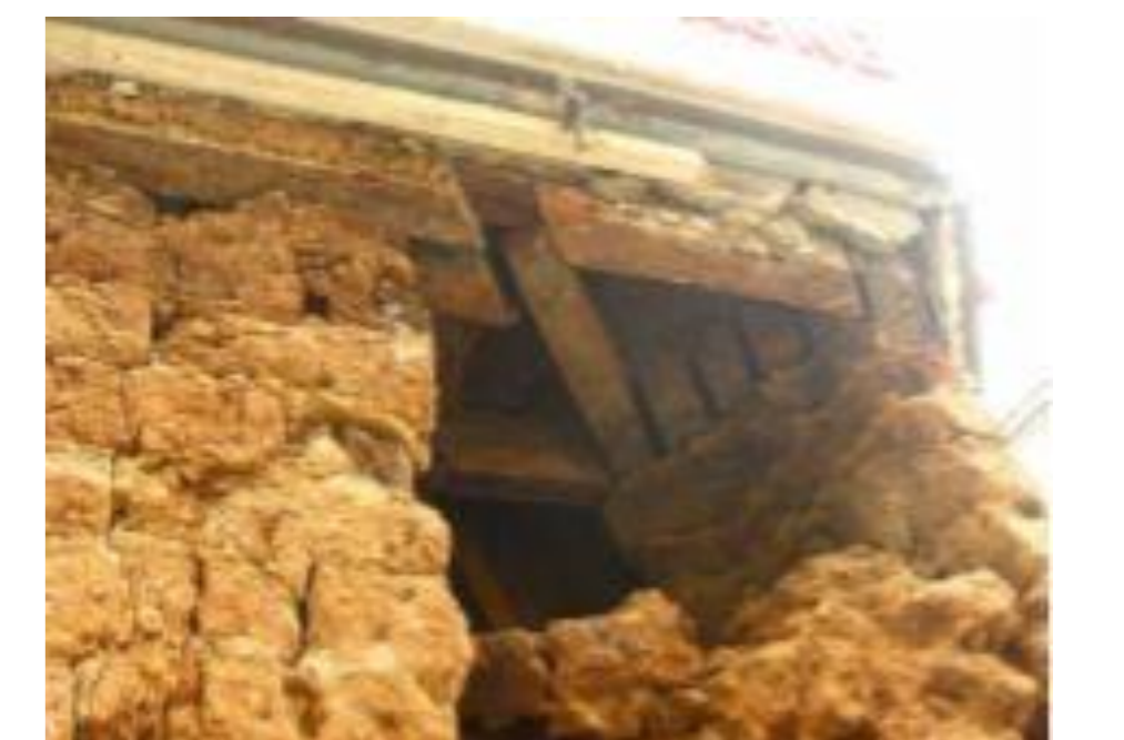
Traditional adobe construction
