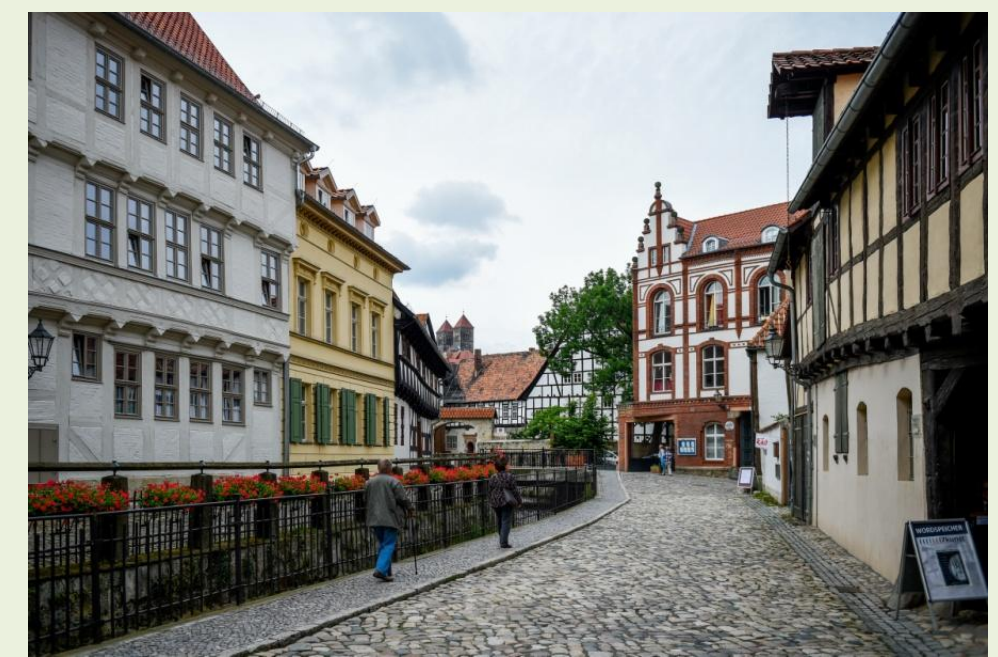
Comprehensive modernisation measures created new apartments and helped develop the Old Town into an attractive residential location. The former barn to the right is now in use for cultural purposes.
