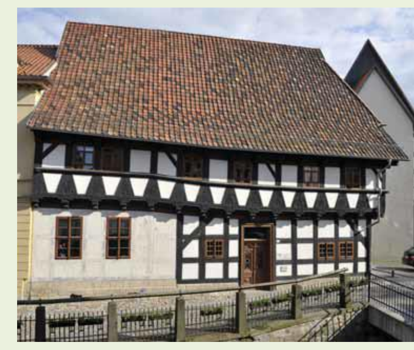
...and after refurbishment. Rich fan rosette carvings on three sides
