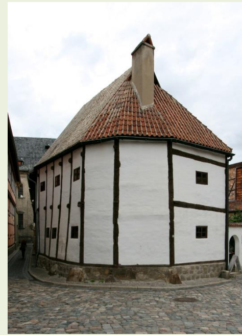
One of the oldest timber-framed houses in Quedlinburg; built in 1347 in the so called „post and beam“ construction. The posts reach from the bottom sill to the roof in one piece.
