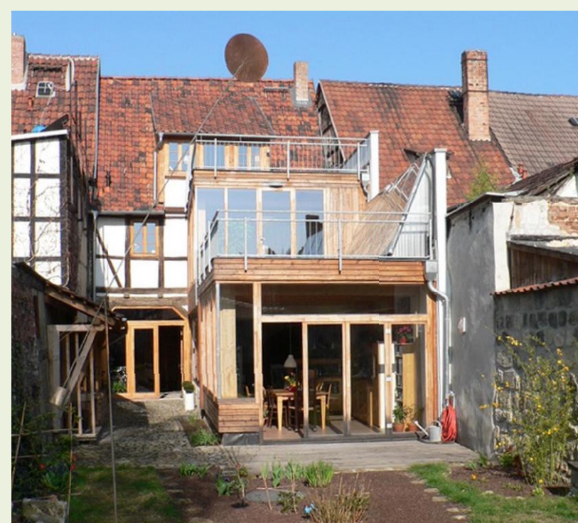
In accordance with monument conservation authorities; generous lighting on the far side of the street allows modern living standards in historic framework houses
