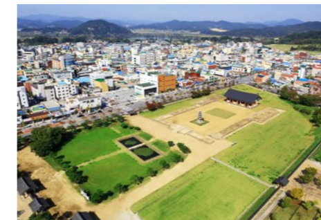
<Photo 5> Bird View of Jeongnimsa Temple Site xiii
