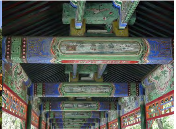
The Summer Palace after its renovation
