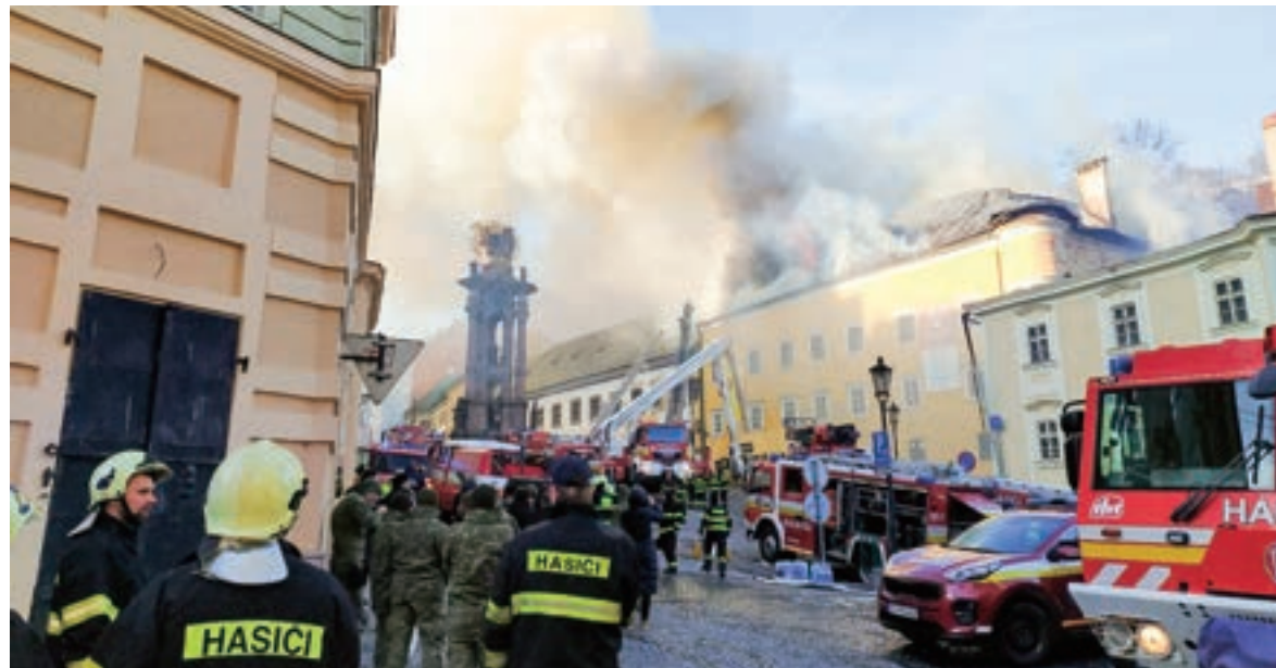
Flames are consuming the roof the Bergerricht House (roof of the Szinyay House already burnt)
