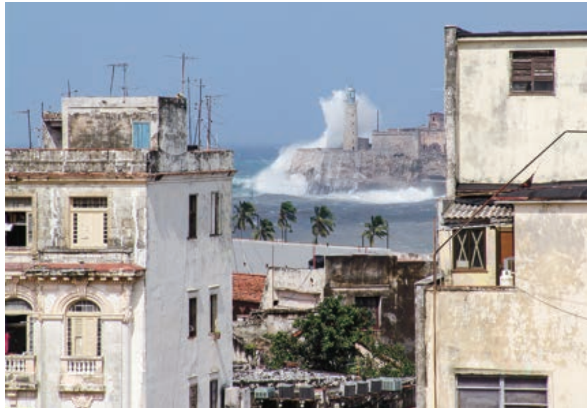
Hurricane damage is visible with Castillo de los Tres Reyes del Morro in the background.
