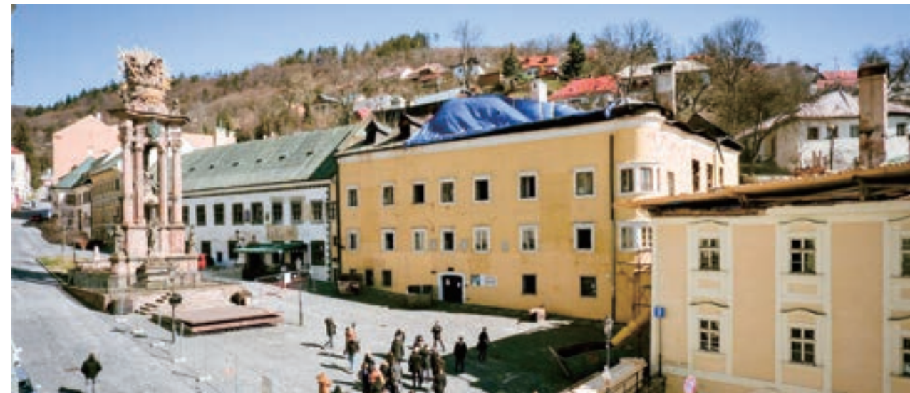
Members of the Government inspect the damaged houses during their meeting in Banská Štiavnica
